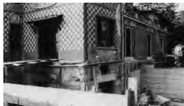
Excavation for the new de Nobili kitchen and terrace.
